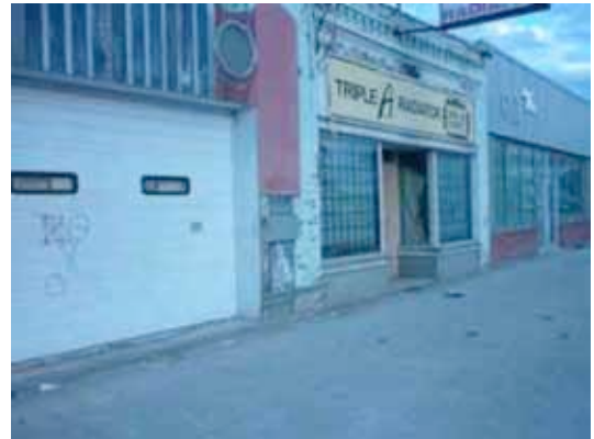
Boarded up businesses on Main Street in the North End
