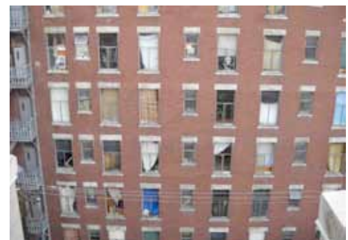
SRO Hotel in the DTES Photo credit: Fred
