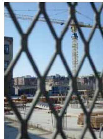
Private condominium development, outskirts of Parkdale Photo credit: Terence
